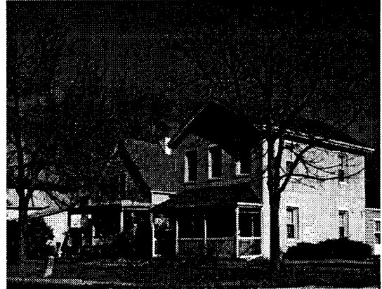
These structures are good examples of appropriate windows and doors because of their vertical proportions.
