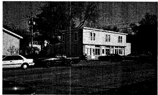
The older commercial structures have a zero setback from the property line, which is typical and appropriate.
