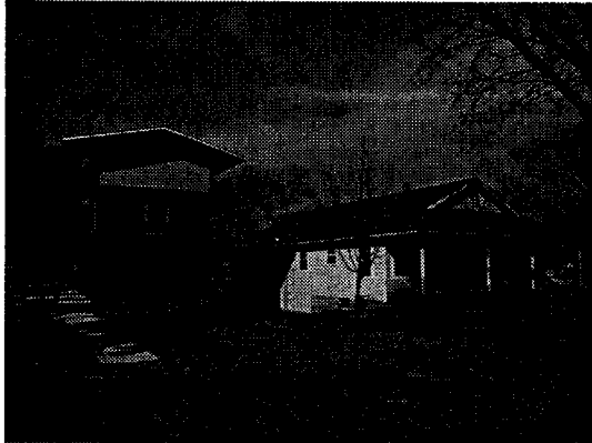
The structure on the left is an inappropriate response to " Building Masses and Spaces " because it is significantly setback further from the street than adjoining structures.
